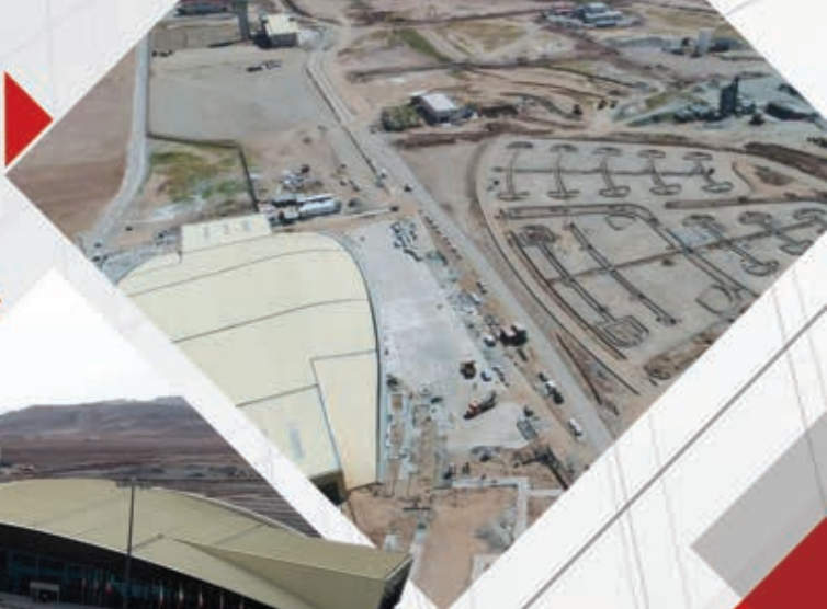
Maku Airport installations and landscaping
